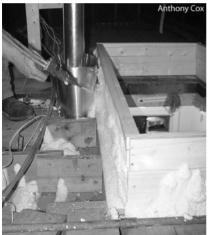
**Two-part foam:** A contractor air-seals around an attic hatch dam with two-part spray foam.
