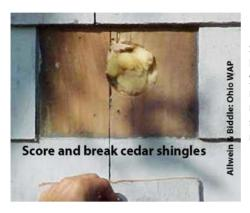
Score and break a shingle: If the shingles are flexible, you may be able to remove nails. However, usually you must score and break the shingle, and then later facenail it back in place.
