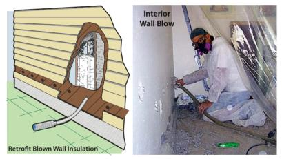
**Tube-filling walls:** perform this method indoors or outdoors. Tube-filling is the preferred wall-insulation method because it achieves a uniform coverage and density.
