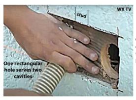
**One hole fills two cavities:** Use a pattern to mark the rectangular hole.
