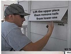
Lift the upper piece: Remove the nails that you expose from the piece below the one you unzipped.
