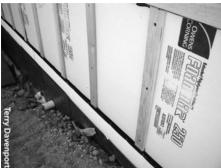
Foam sheathing with battens: Oneby-four battens are applied to 4 inches of foam board on the exterior to provide a fastening strip for siding and trim.
