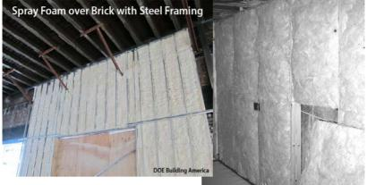
**SPF insulates, seals, and reinforces brick wall:** In this installation, open-cavity spray foam performs three separate functions.
