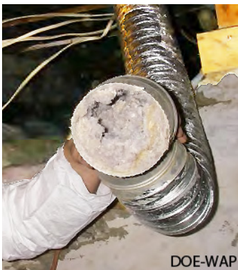
Lint collection: After years of operation, lint coats flexible pipe and eventually blocks the airway.
