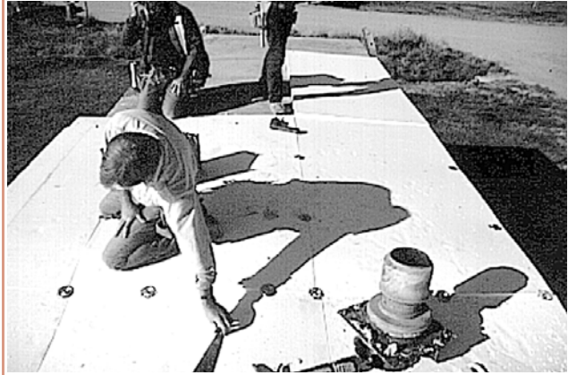
Figure 10-17 Rooftop Insulation
