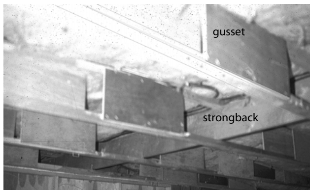
Figure 10-3 Bowstring Trusses
