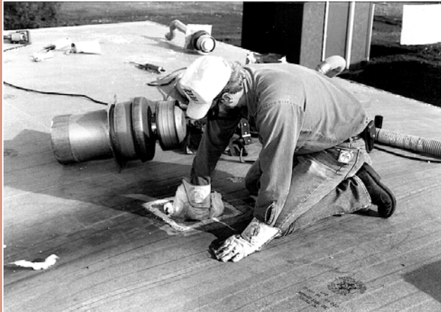
Figure 10-9 Protecting the Chimney
