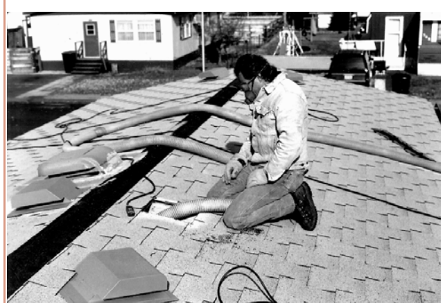
Figure 10-16 Insulating Shingled Double-wide Roof Cavities
