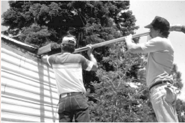
Figure 10-12 Blowing Insulation through the Roof's Edge
