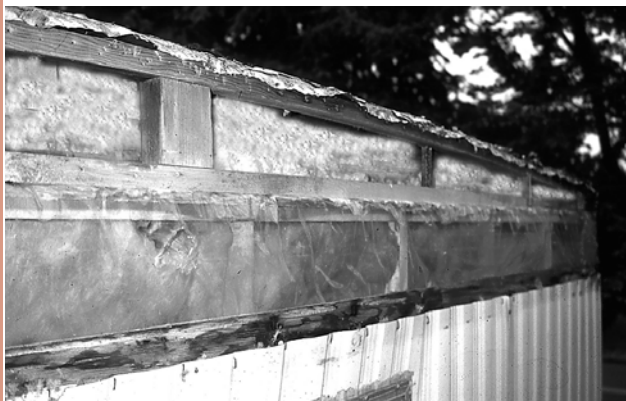
Figure 10-15 Insulating a Single-Wide from the End Wall
