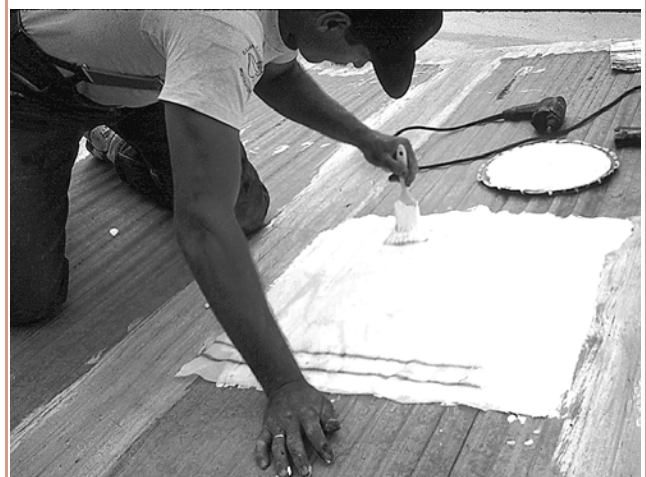
Figure 10-7 White Latex Roof Coating
