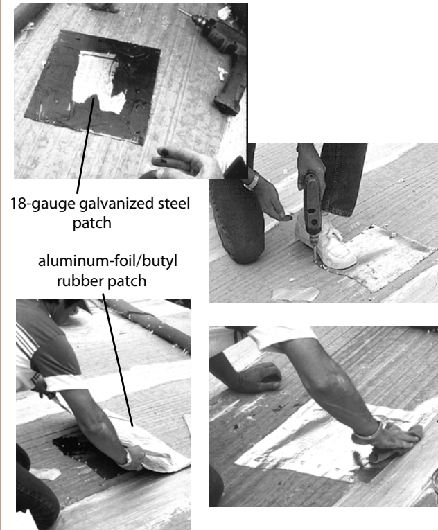
Figure 10-8 Patching a Large Hole
