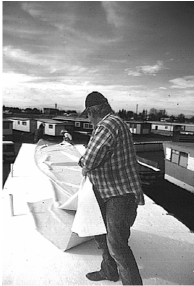
Figure 10-18 Covering the Insulation with Rubber Roofing
