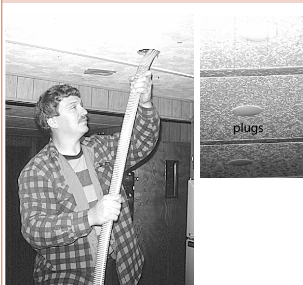
Figure 10-13 Blowing through the Ceiling Indoors
