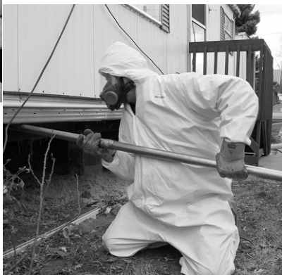
Patching a flexible belly: The technician uses both adhesive and stitch staples to fasten a patch.
