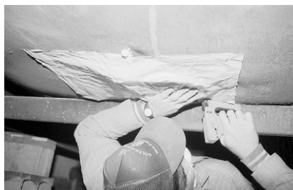
Patching a flexible belly: The technician uses both adhesive and stitch staples to fasten a patch.
