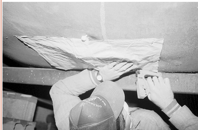
Figure 7-6 Outward Clinch Stapler
