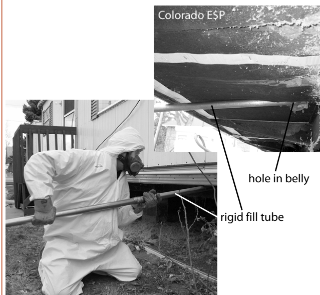
Figure 7-12 Blowing Floor Insulation
