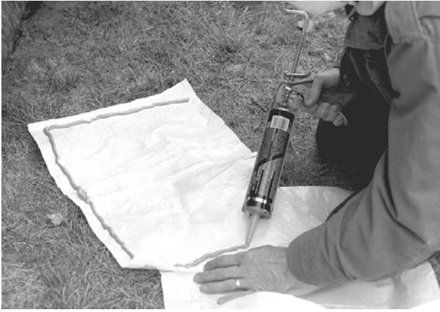
Figure 7-5 Underbelly Patch
