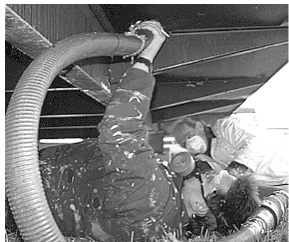
Figure 7-7 Blowing Floors from Underneath
