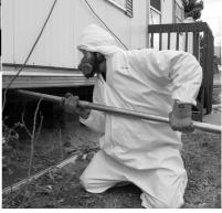
Blowing a floor through the belly: The contractor inserts a rigid fill tube through the belly to blow insulation into the floor cavity and underbelly.
