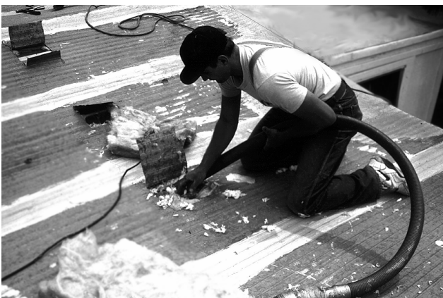
Figure 1-15 Filling Roof Cavities with Blown Insulation
