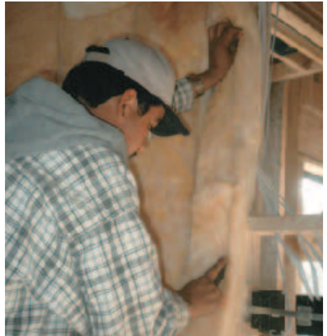
Figure 2. To achieve the required tight fit, batts are trimmed to the required height and width in place. Each batt is pushed tight to the sheathing, then pulled forward until it's flush with the stud faces. On inspection tours, the author checks for exposed stud shoulders and makes sure batts have been split around wires as needed.
