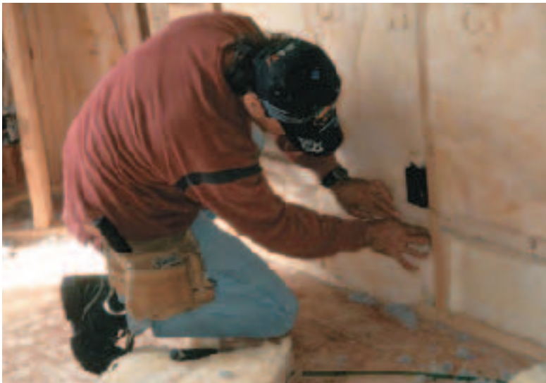
Figure 2. To achieve the required tight fit, batts are trimmed to the required height and width in place. Each batt is pushed tight to the sheathing, then pulled forward until it's flush with the stud faces. On inspection tours, the author checks for exposed stud shoulders and makes sure batts have been split around wires as needed.
