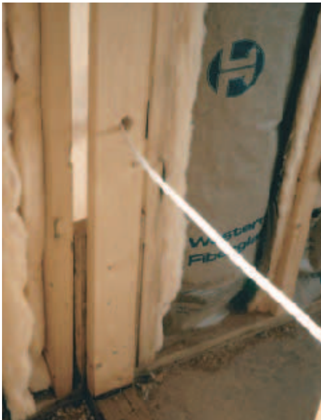
Figure 3. Framers often leave spaces blocked off that are hard or impossible to insulate. Left, the intersection between an interior and an exterior wall can be reached only through a small gap. Above, a wood I-joist has been hung out over the top plate to serve as a nailer for the ceiling drywall, completely blocking access to the band joist. (For the correct detail in this area, see Figure 6.) In both photos, the kraft-faced batts have been jammed into place with no effort to achieve a proper fit.
