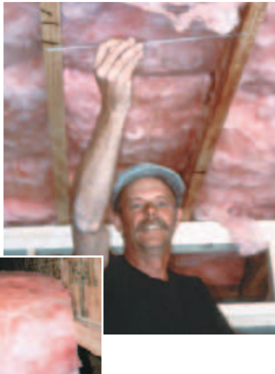
Figure 12. The author uses 16-inch-wide commercial batts to insulate engineered floors. He recommends wire batt hangers (left) to hold the batts tight to the floor sheathing. Standard-width batts don't fit snugly between the thin webs of wood I-joists (below).
