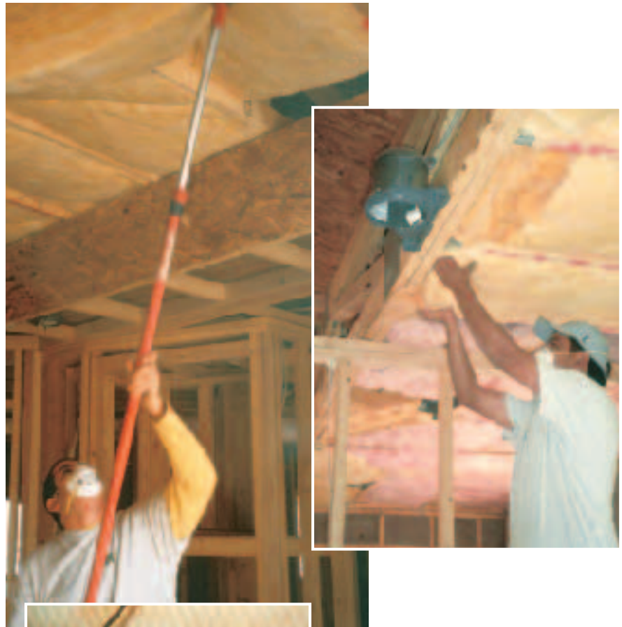
Figure 8. The author’s crew uses toro poles with pronged ends to place batts in high ceilings (left). To reduce convection and infiltration losses, batts should be pulled down to make contact with the ceiling drywall (above).
