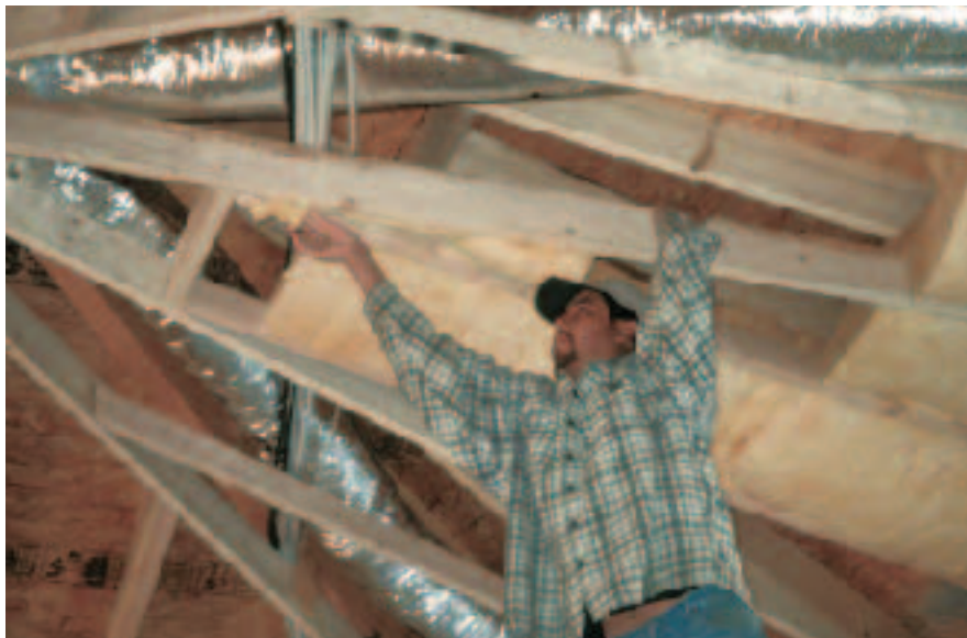
Figure 7. Low “Santa Fe” attics like this one don’t leave room for blown-in products. Instead, carefully fitted batts are installed between the bottom truss chords.
