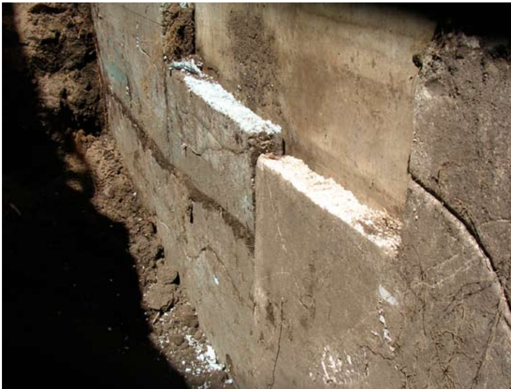
Figure 2. XPS and EPS below grade insulation
