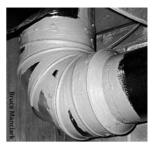
Sectioned elbows: Joints in sectioned elbows, known as gores, are usually leaky and require sealing with duct mastic.
