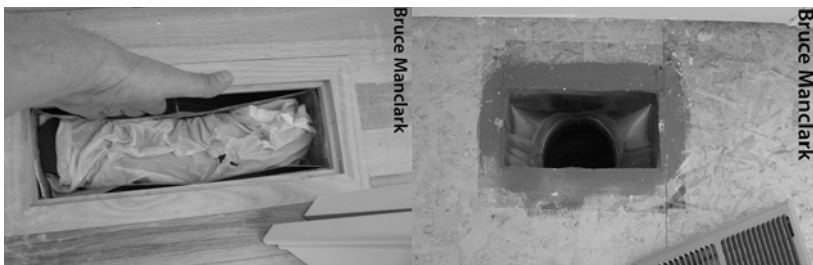
Sealing register boots: Seal between the boot and floor. Seal joints inside the boot.
