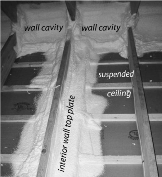
**Sealing structural suspended ceilings:** Two-part foam air seals an interior wall top plate and the wall cavity between the ceiling and roof deck.
