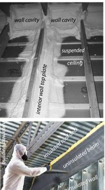
Sealing structural suspended ceilings: Two-part foam air seals an interior wall top plate and the wall cavity between the ceiling and roof deck.
