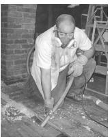
**Finished attic floor:** Find the large air leaks underneath the flooring and seal them before insulating the space between the joists.
