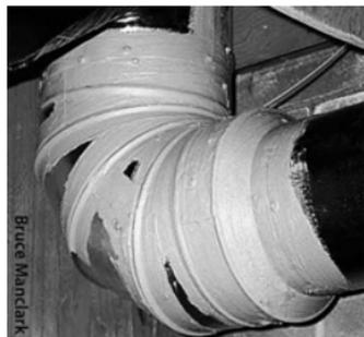
**Plenums, poorly sealed to air handler:** When air handlers are installed in tight spaces, plenums may be poorly fastened and sealed. Cutting a hole in the duct may be the only way to seal this important joint.
