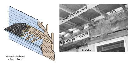
**Porch air leakage:** Porch roof cavities often allow substantial air leakage because of numerous joints, and because there may be no siding or sheathing installed in the wall behind the roof and ceiling.
