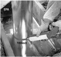
Sealing manufactured chimneys: When installing retrofit insulation in addition to air sealing, install a shield on top of the air seal that extends above the level of the new insulation.
