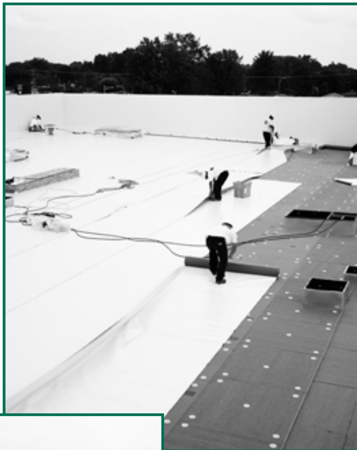
Above: Figure 4: Workers lay membrane over foam insulation at Brett Favre's Steakhouse, Green Bay, WI. (Photo courtesy Johns Manville).
