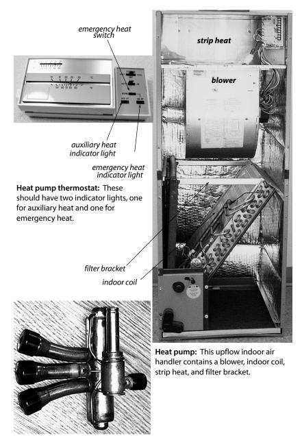
**Reversing valve:** The outdoor unit contains a reversing valve installed near the compressor.
